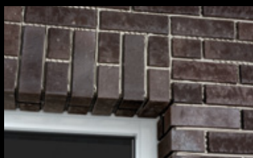
Window lintel perfectly replicated with angles.
