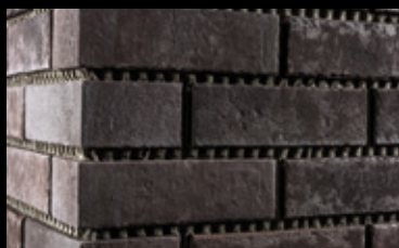
The finished surface. Grouting can be done after the appropriate drying time.
