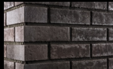
The finished joint pattern. Full masonry stretches are grouted at one go.
