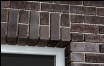
Window lintel perfectly replicated with angles.
