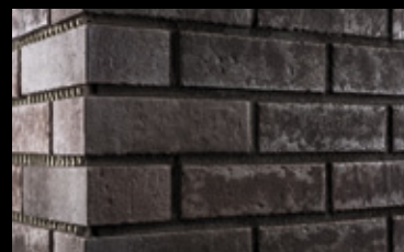
The finished joint pattern. Full masonry stretches are grouted at one go.
